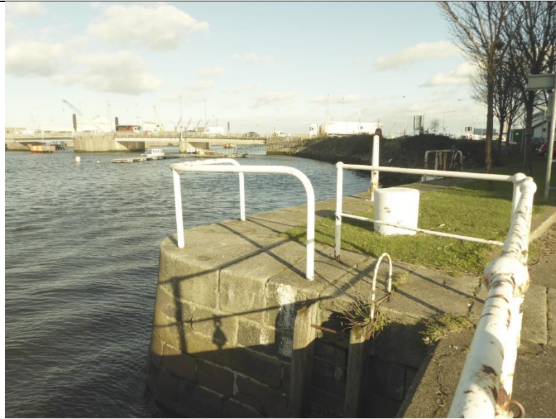
Look east at the stone quay showing the railings, wooden ladder and mooring stone
