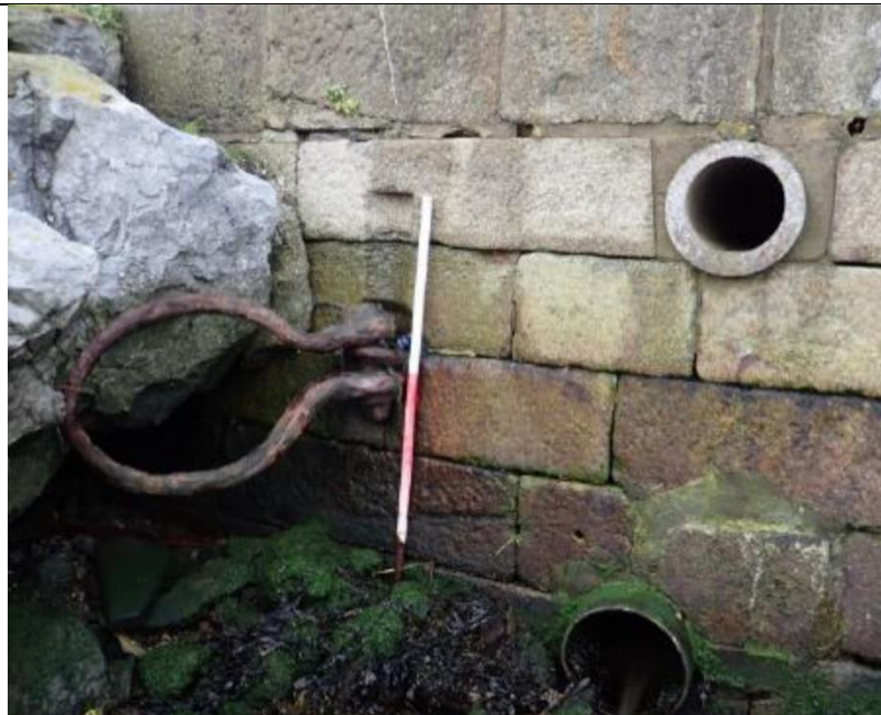
Historic stone quay: Mooring Ring and modern outfalls facing south
