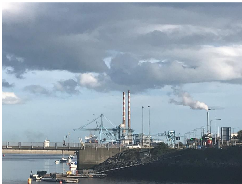
Rock armour and reclaimed land facing east taken from Britain Quay
