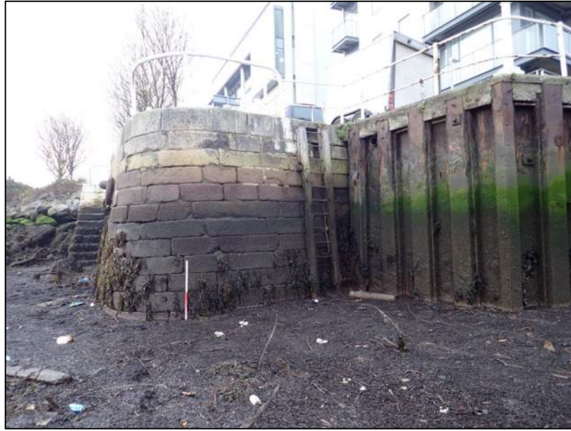
Plate 11: East-facing view of rounded corner of a historic masonry quay at Thorncastle Court (1m scale). Note Larson pile quay obscures much of western faced of the structure.
