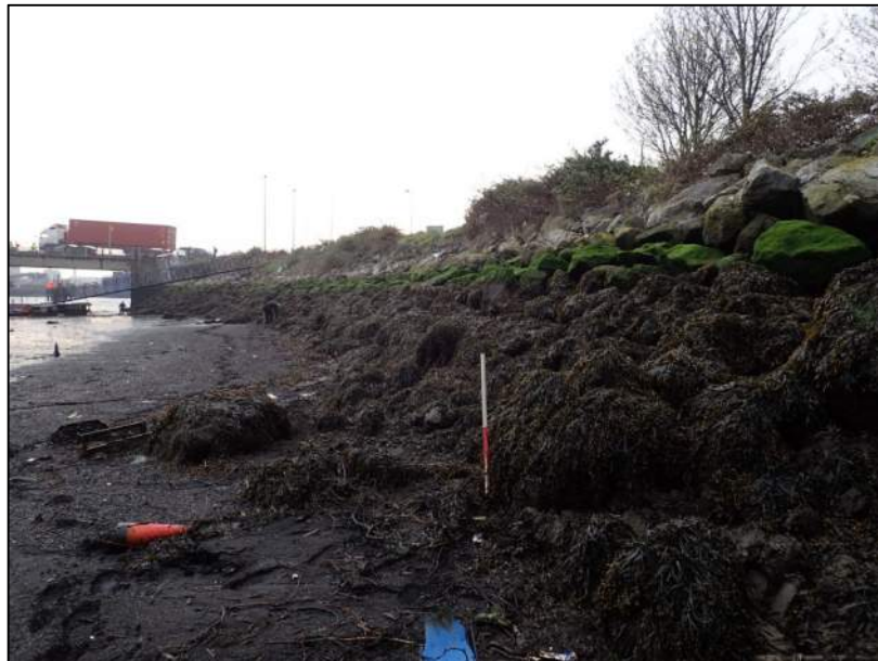
Plate 12: East-facing view of rock-armour that delineates much of the south side of the River Liffey on upstream side of the East Link Bridge. Note the placement of which obscures the true extent of the historic masonry quay at Thorncastle Court (1m scale).
