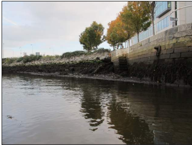
Plate 15: East-facing view of masonry quayside with flight of river-access steps in background. Note rock-armour obscuring original line of quayside.
