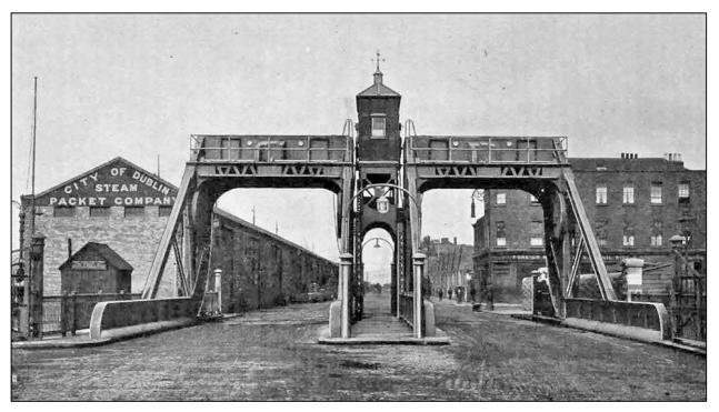
**1913** View from west towards City end showing both bridges open for road traffic. The motors which powered each of the bridges are visible half-way along each gantry in front of the overhead counterweights. (*Griffith 1913*)
