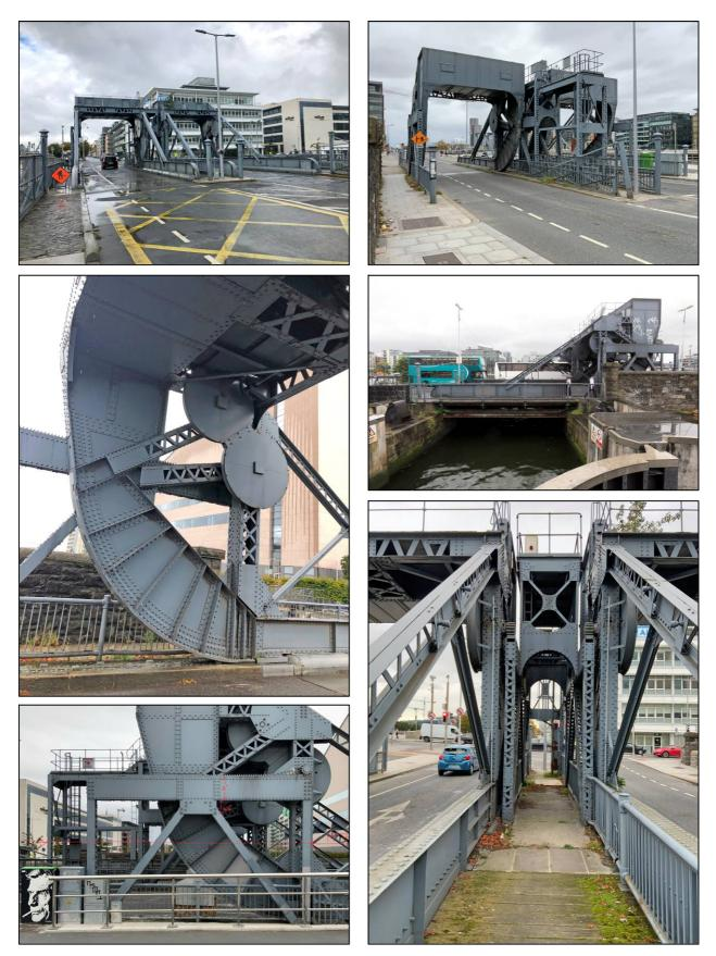
Fig 4.3 Contemporary photographs of Scherzer bridges over Royal Canal. *Top left* - From east; *Top right* - From west; *Middle left* - Quadrant roller; *Middle right* - From north; note lock gate winches in front. *Bottom left* - Track along winch bridge travels. *Bottom right* - Control cabin platform from east.
