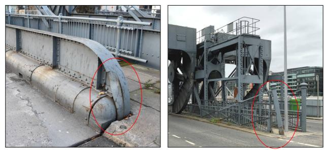
Fig 4.5 Traffic impact damage. *Left:* Bent flange on main girder at east end of Outer Bridge. *Right:* Damaged traffic control gatepost at west end of Inner Bridge.
