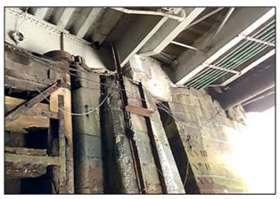
Lock gate on east side. Note the vertical slot at right for timber baulks to cut the channel off from the river.
