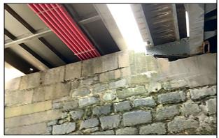
Looking W showing one of the 2019 spans carried over the top of the canal's side wall. By contrast, the end of the Outer Bridge (*at right*) is let into its top.
