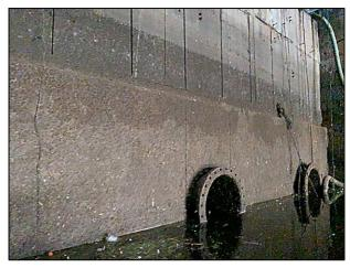
Concrete wall across lock chamber, with drainage pipes along bottom.
