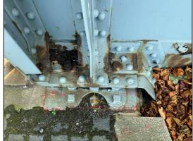
Fig 7.5 *Left:* Incomplete spur gear on Outer Bridge. Note also bent flange on cross member due to strike from a high load. *Above:* Minor rusting on flange plates.
