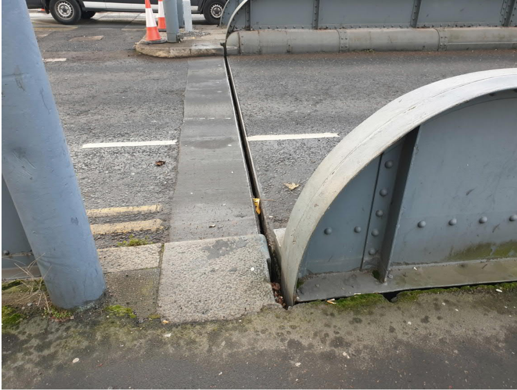
Figure 7: Expansion joint detail in the Scherzer bridges
