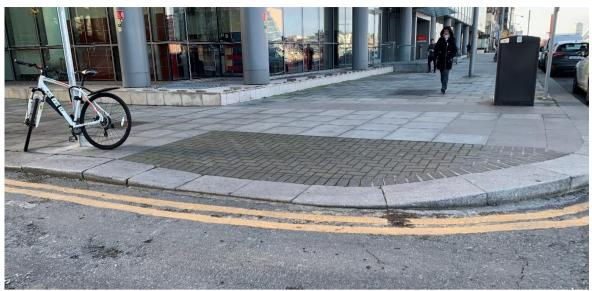
Cobble lock used in lieu of blister tactile paving at uncontrolled crossings
