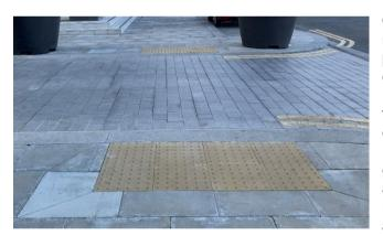
Only one minor access street was noted on the south quays where pedestrians have not been given crossing priority over it. This is reinforced through the presence of tactile paving despite the continuation of pavement materials. It is recommended that priority be given to pedestrians across all accesses to reduce the level of uncertainty over priority on what appears to be footpath.
