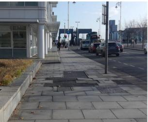
Cobbles and red paving on the campshire [left] and poor asphalt repairs [right]
