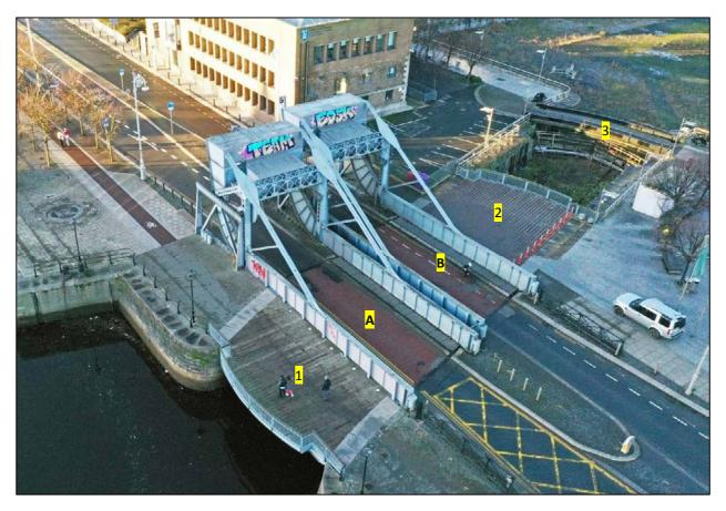
Fig 6.9 Aerial view of modern bridges over the entrance to George's Dock, from SE, 2021. *Key:* A - Outer Scherzer; B - Inner Scherzer; 1 - Modern foot bridge; 2 - Modern footbridge; 3 - Vehicle access bridge.
