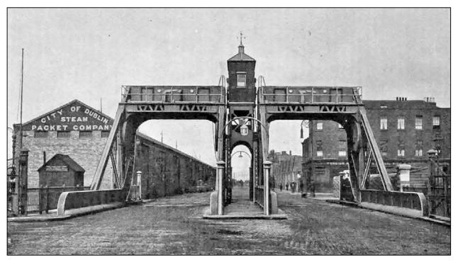
**1913** View from west towards City end showing both bridges open for road traffic. The motors which powered each of the bridges is visible half-way along each gantry in front of the overhead counterweights. (*Griffith 1913*)
