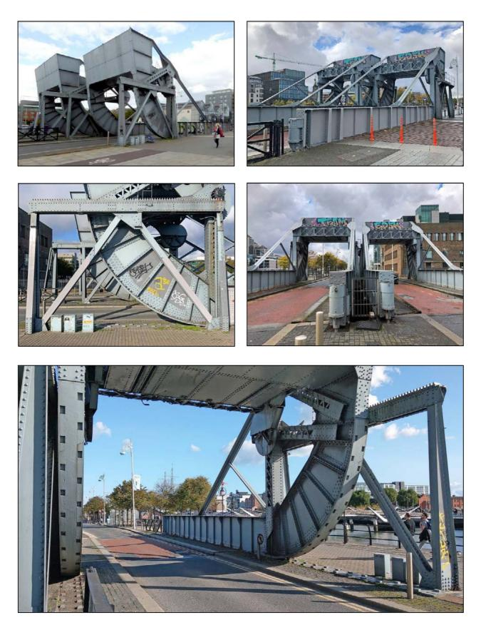
Fig 7.3 Contemporary photographs of Scherzer bridges at George's Dock. *Top left* - From SW; *Top right* - From NE; *Middle left* - Rack and pinion (at right end of rack); *Middle right* - Air buffers at lifting end of spans. *Bottom* - Quadrant rollers and toothed track plates along which they travel.
