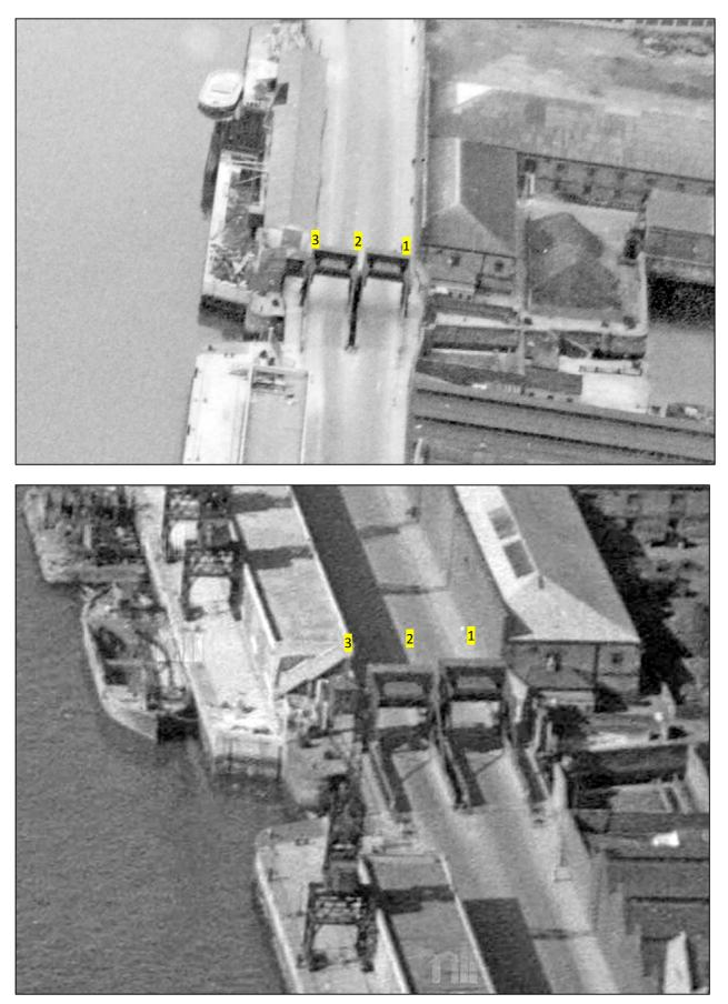
Fig 6.8 Aerial views of Scherzer bridges over entrance to George's Dock, from east. Top: 1949 view (Britain from Above, XAW027127). Bottom: 1955 view (National Library Ireland, Morgan Aerial Photographic Collection). Key: 1 - Inner Bridge, 2 - Outer Bridge, 3 - Overhead control cabin.
