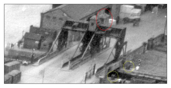
Enlarged aerial view from NE, 1950. The original control cabin platform has now been extended towards the City end and a second cabin erected (circled in red). Note also the two winches (in yellow) which were installed to work the timber lock gates when the Inner Bridge was erected. They still exist but are no longer in use. (*Britain from Above, XAW032929*)
