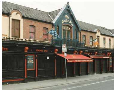
Proposal to knock down Drake Inn and build flats was rejected
